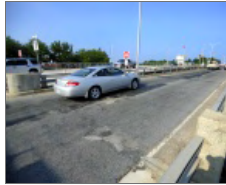
Causeway bridge work to start soon
